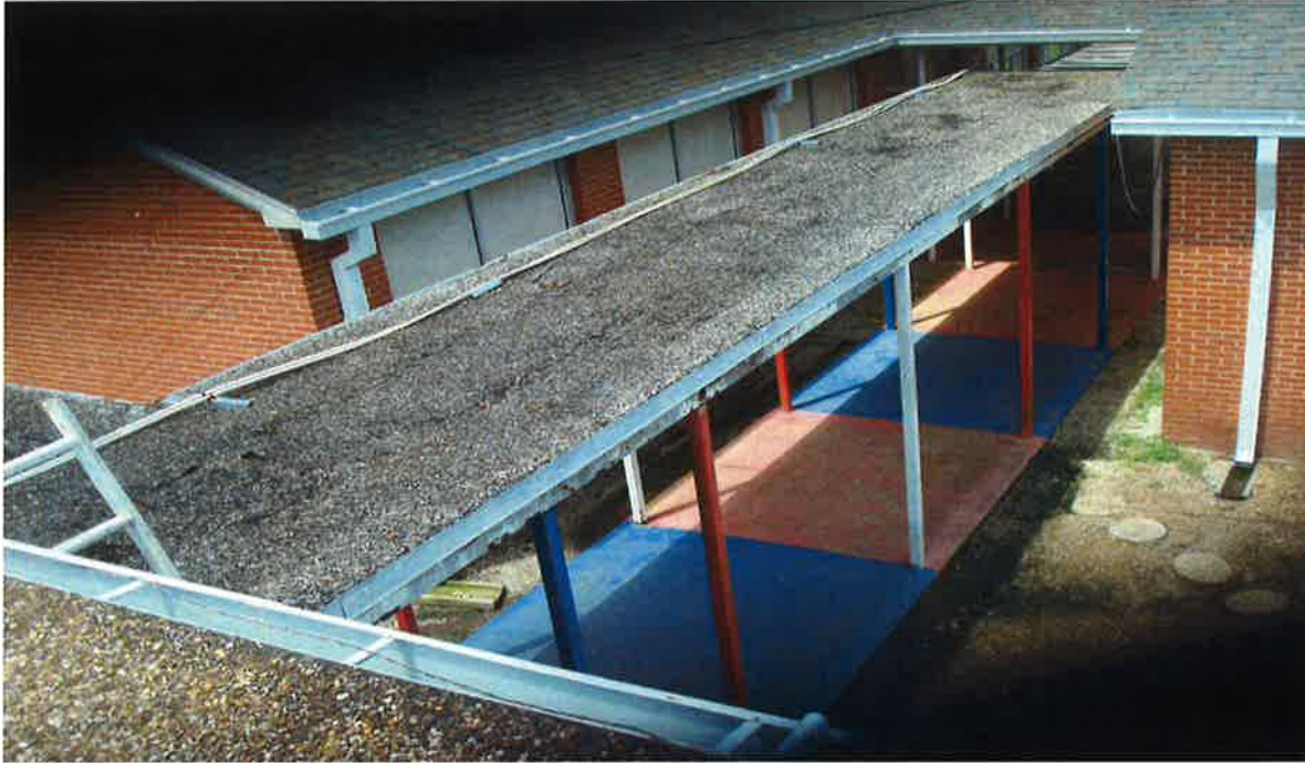
Built Up Roofing Homogenous Area (HA) (123-06)
