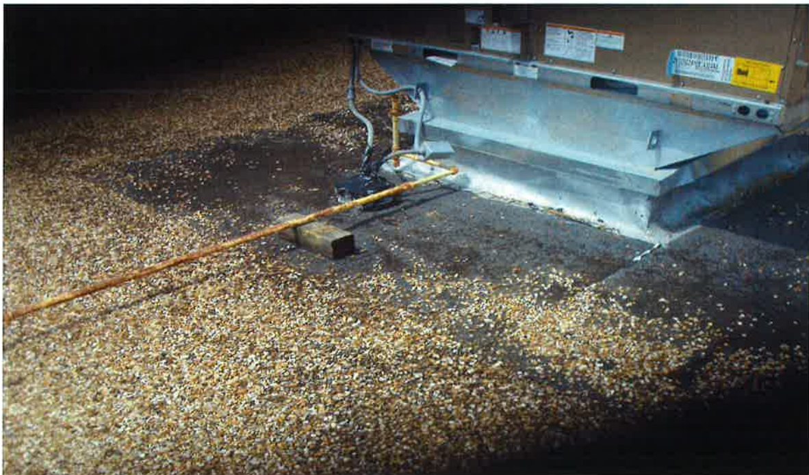
Roof Penetration Flashing Homogenous Area (HA) (123-03)
