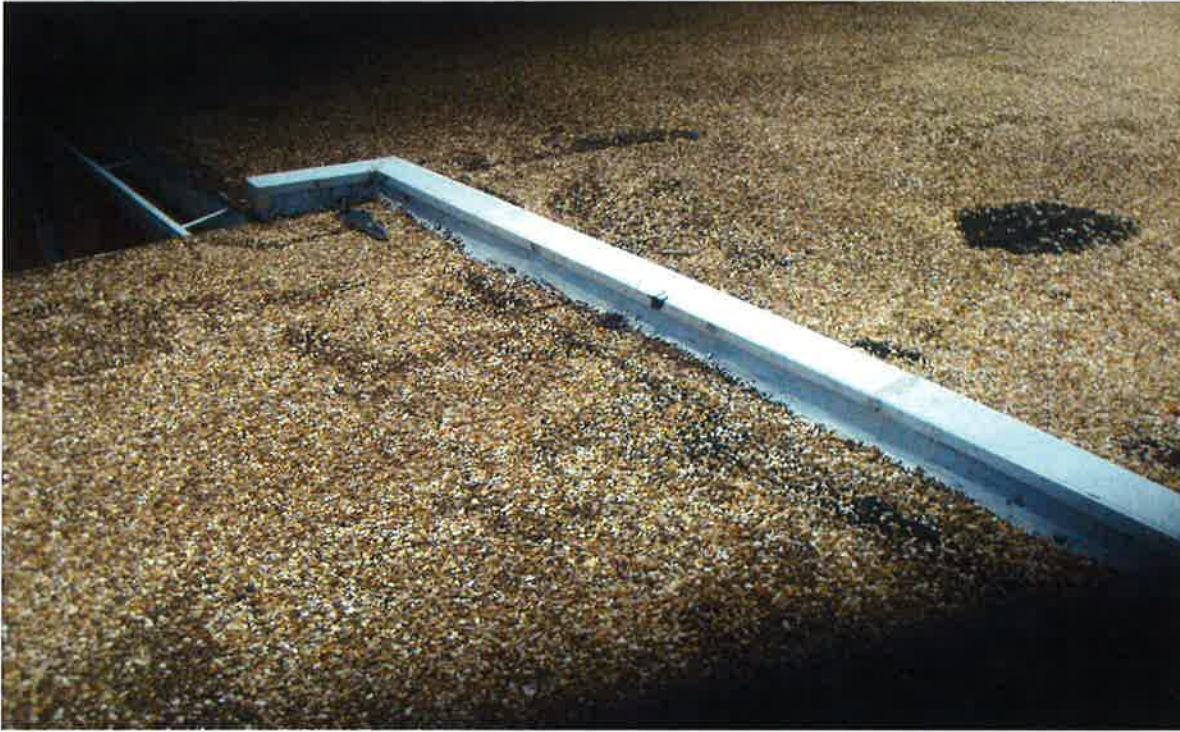
Roof Expansion Joint Homogenous Area (HA) (123-05)
