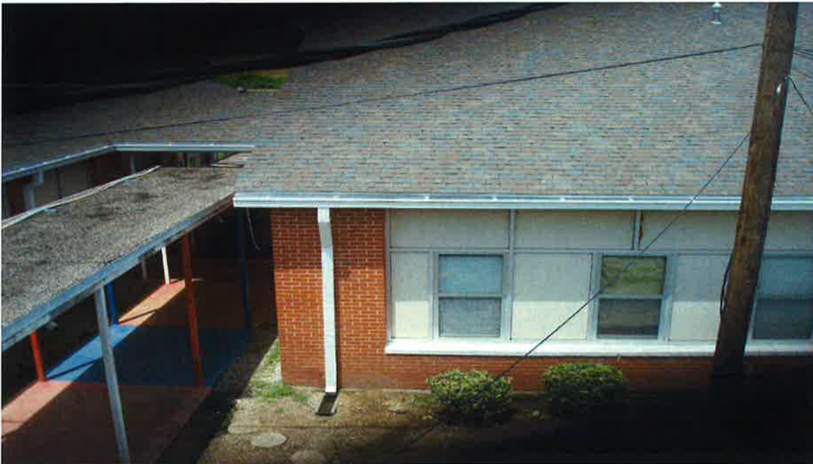
Roof Single Homogenous Area (HA) (45-01)
