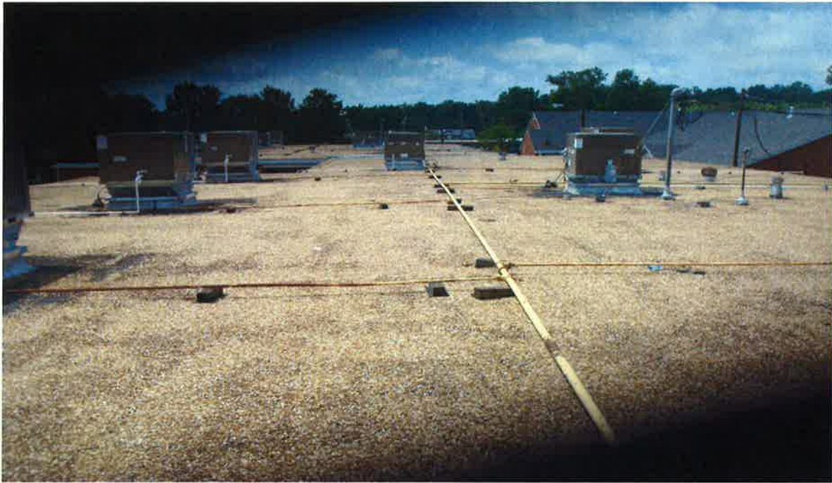
Built Up Roof Homogenous Area (HA) (123-01)
